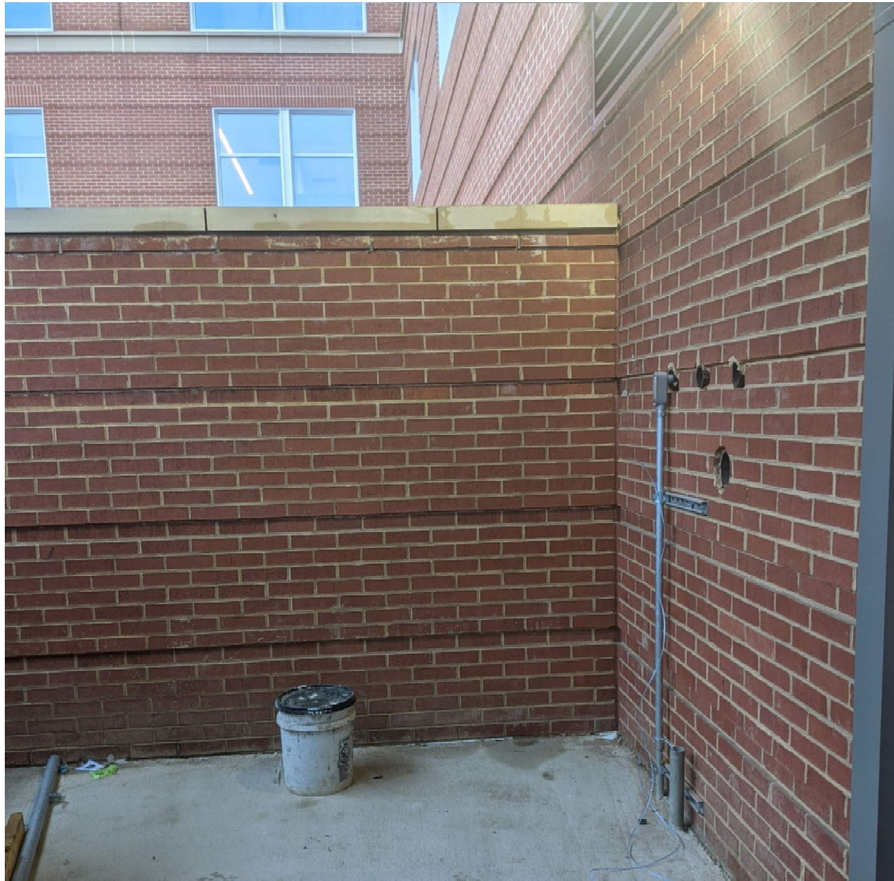
EXTERIOR CONDITIONS – SCREEN WALL AREA
