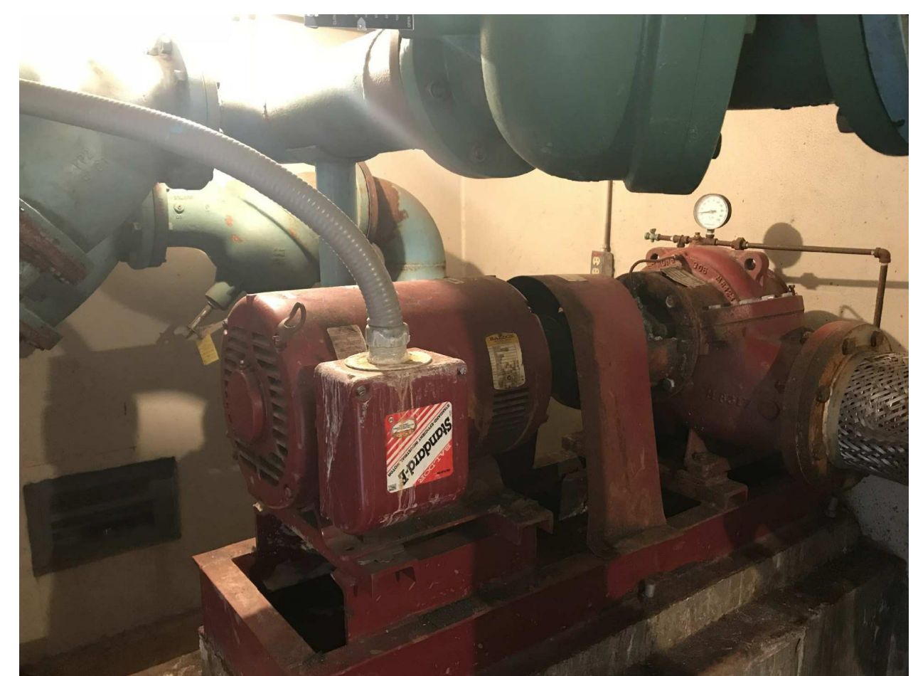
PHOTO OF EXISTING CWP-5 TO BE REPLACED BELOW TOWER
