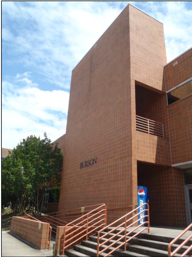
NO. 39 – NORTH ELEVATION – EAST EXTERIOR STAIRWELL
