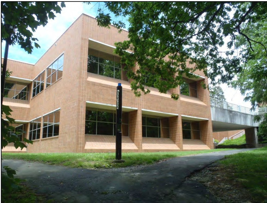
NO. 28 – PARTIAL SOUTH ELEVATION
