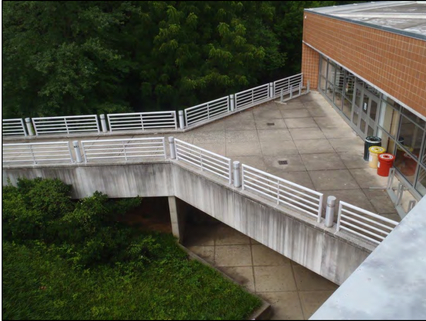
NO. 99 – SECOND FLOOR SOUTHEAST ENTRY PLAZA
