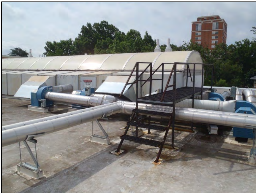
NO. 190 – ROOF VIEWS FROM THE WEST FACE
