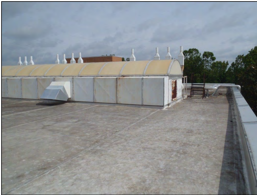
NO. 172 – ROOF VIEWS FROM THE EAST EDGE
