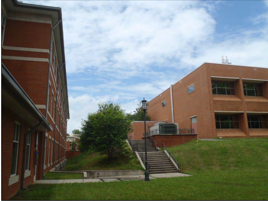
NO. 23 – PARTIAL SOUTHWEST ELEVATION
