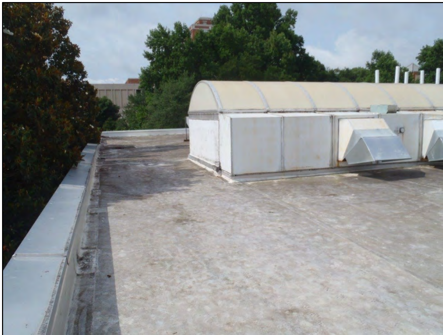
NO. 169 – ROOF VIEWS FROM THE EAST EDGE
