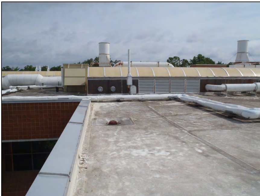
NO. 177 – ROOF VIEWS FROM THE SOUTH FACE
