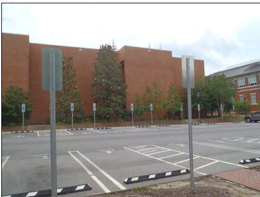
NO. 17 – PARTIAL NORTH ELEVATION
