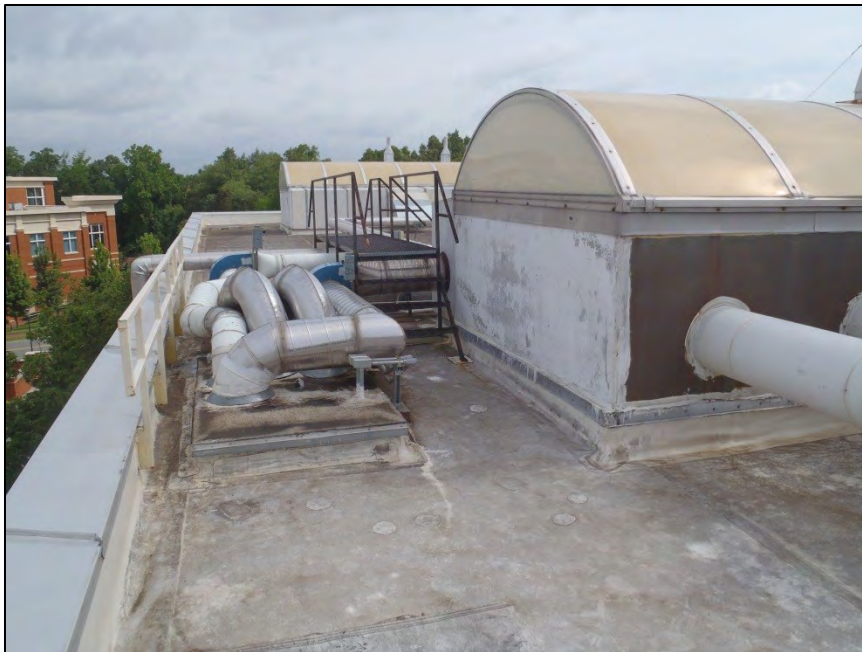
NO. 183 – ROOF VIEWS FROM THE SOUTHWEST CORNER
