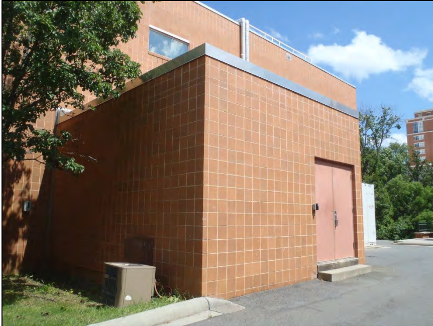
NO. 78 – WEST ELEVATION – BASEMENT ADDITION
