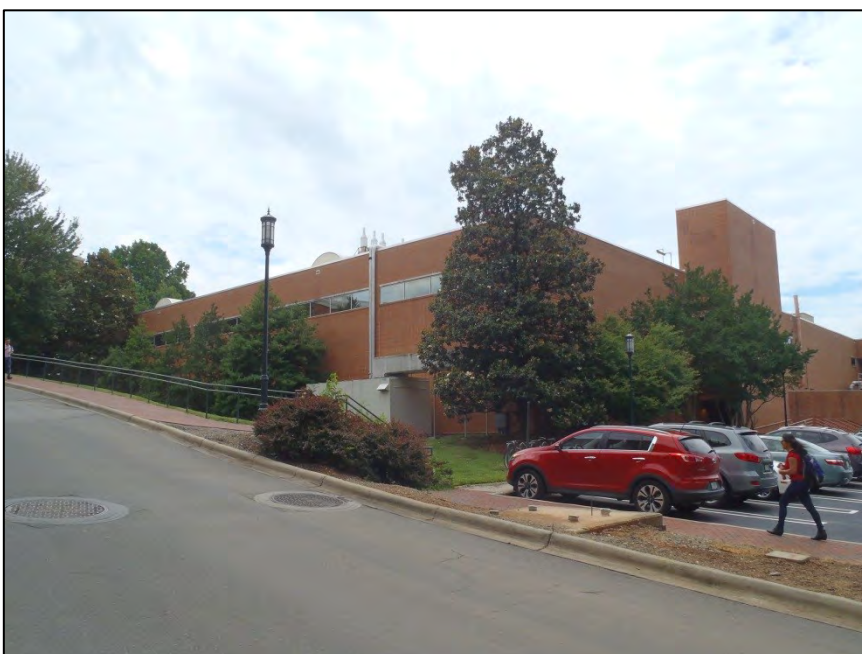
NO. 11 – PARTIAL NORTHEAST ELEVATION
