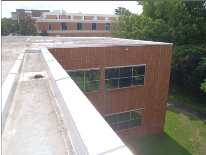
NO. 180 – ROOF VIEWS FROM THE SOUTH FACE
