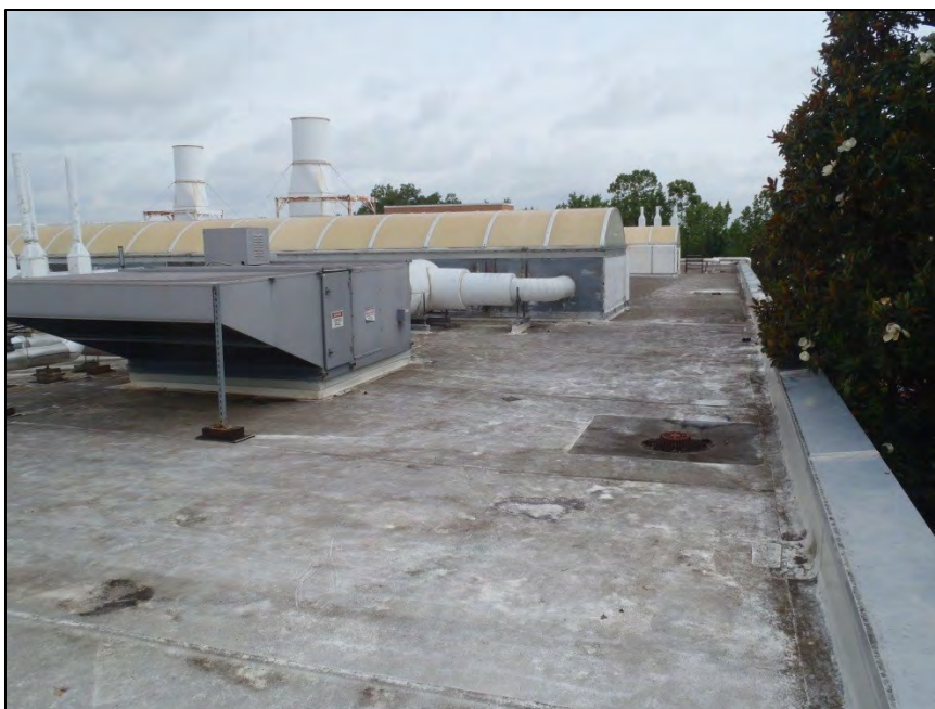
NO. 175 – ROOF VIEWS FROM THE SOUTHEAST CORNER
