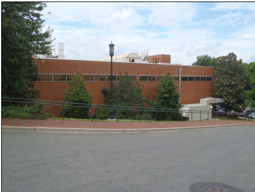
NO. 10 – PARTIAL EAST ELEVATION
