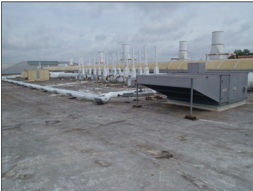
NO. 174 – ROOF VIEWS FROM THE SOUTHEAST CORNER
