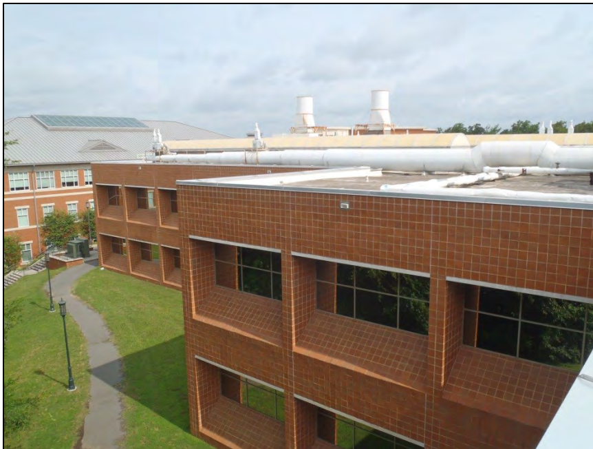
NO. 176 – ROOF VIEWS FROM THE SOUTH FACE
