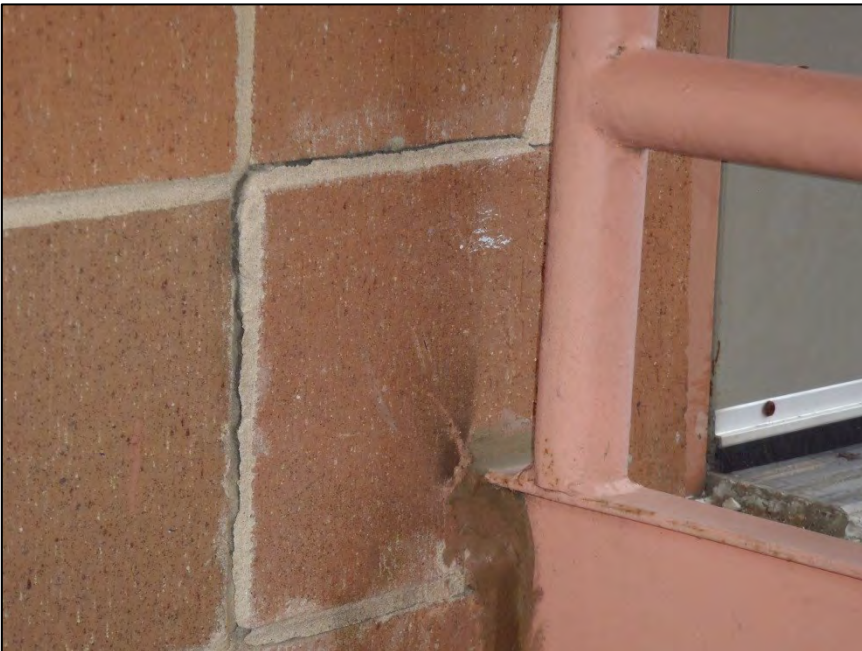
NO. 63 – NORTH ELEVATION AT CENTER EXTERIOR STAIRWELL – DETERIORATED STEEL GIRDER AND SPALLED BRICK VENEER AT BEAM BEARING LOCATION
