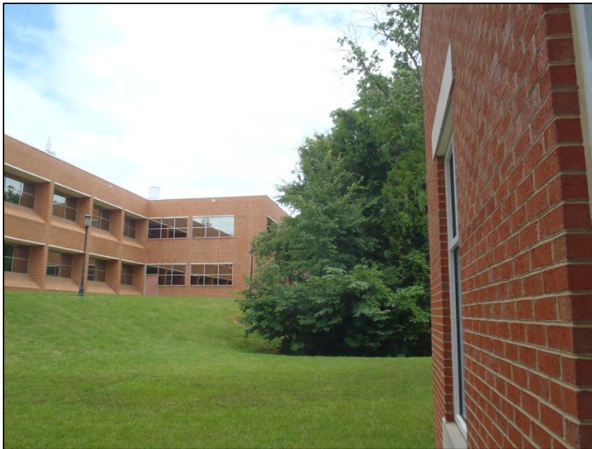
NO. 26 – PARTIAL WEST ELEVATION
