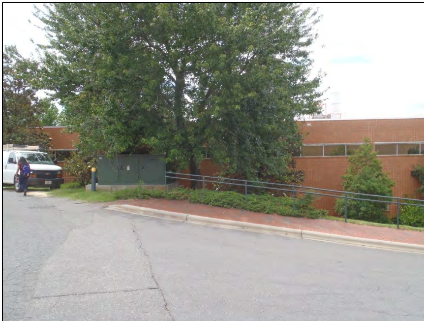
NO. 9 – PARTIAL EAST ELEVATION
