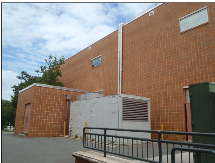
NO. 22 – PARTIAL WEST ELEVATION
