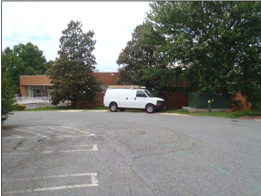
NO. 7 – PARTIAL EAST ELEVATION
