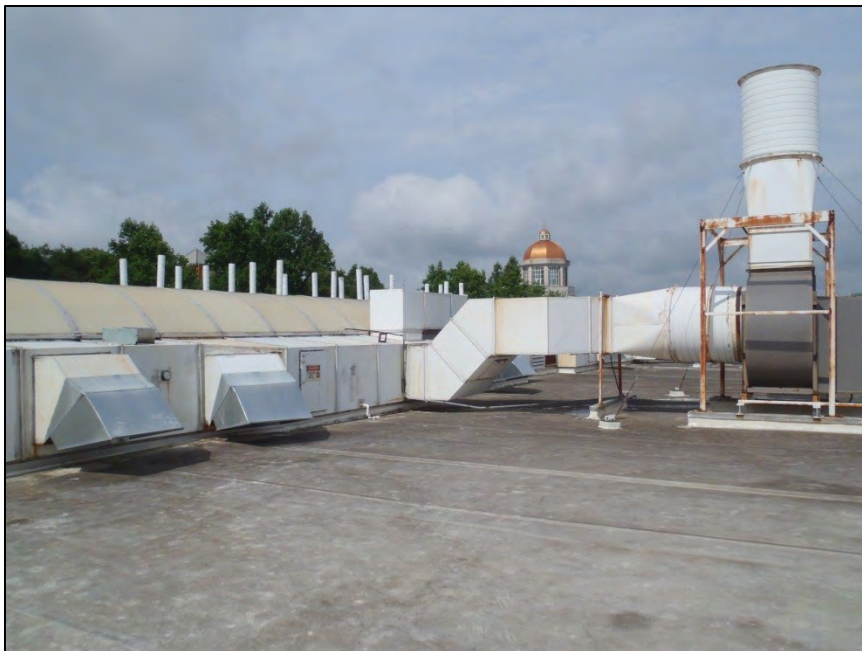
NO. 170 – ROOF VIEWS FROM THE EAST EDGE
