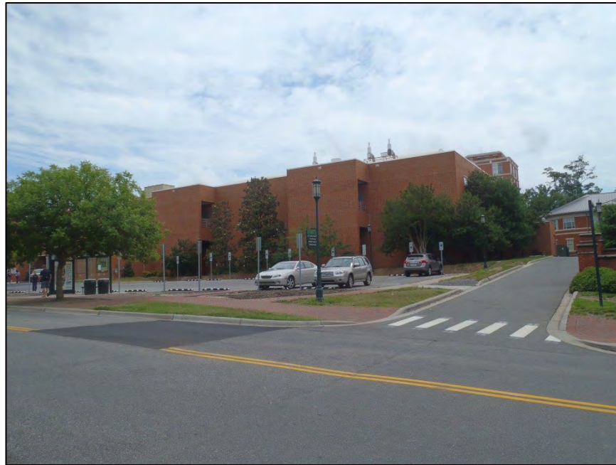
NO. 19 – PARTIAL NORTHWEST ELEVATION
