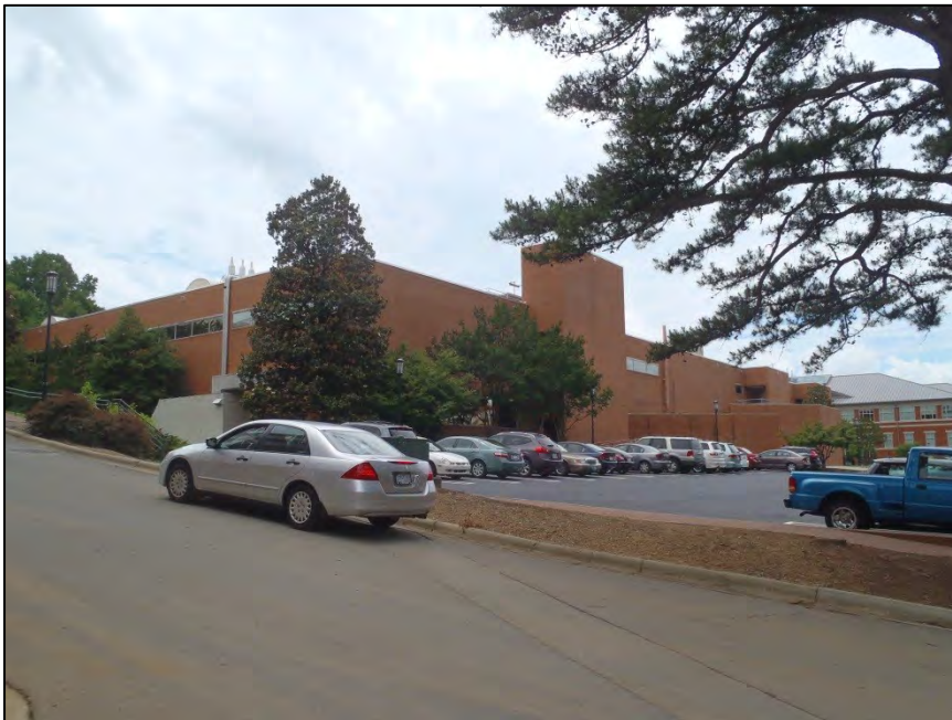
NO. 12 – PARTIAL NORTHEAST ELEVATION
