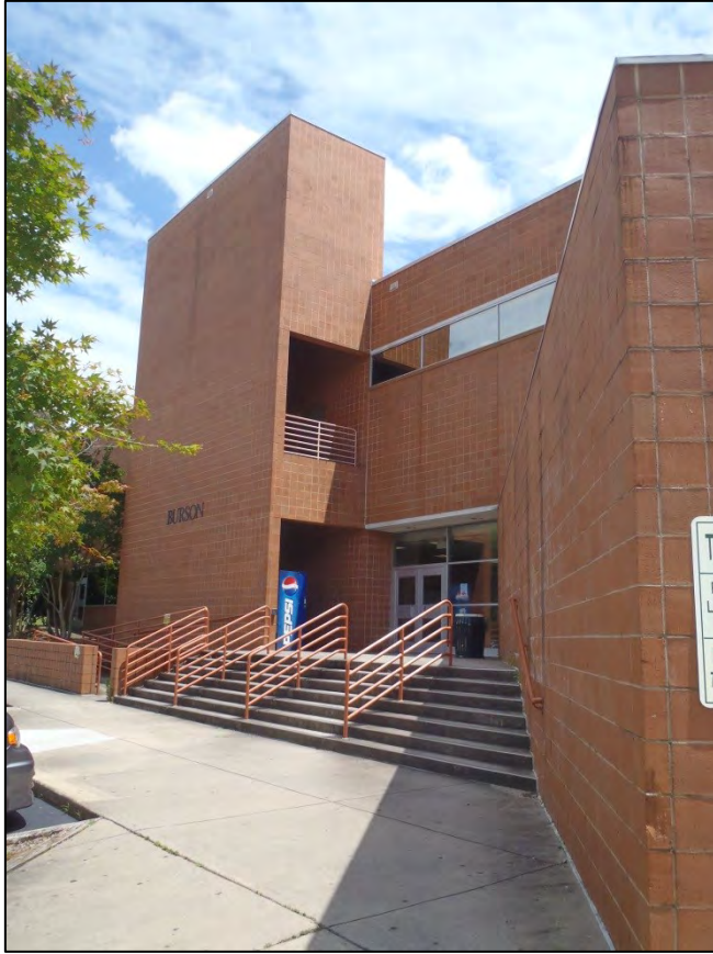
NO. 46 – NORTH ELEVATION AT EXTERIOR SCREEN WALL
