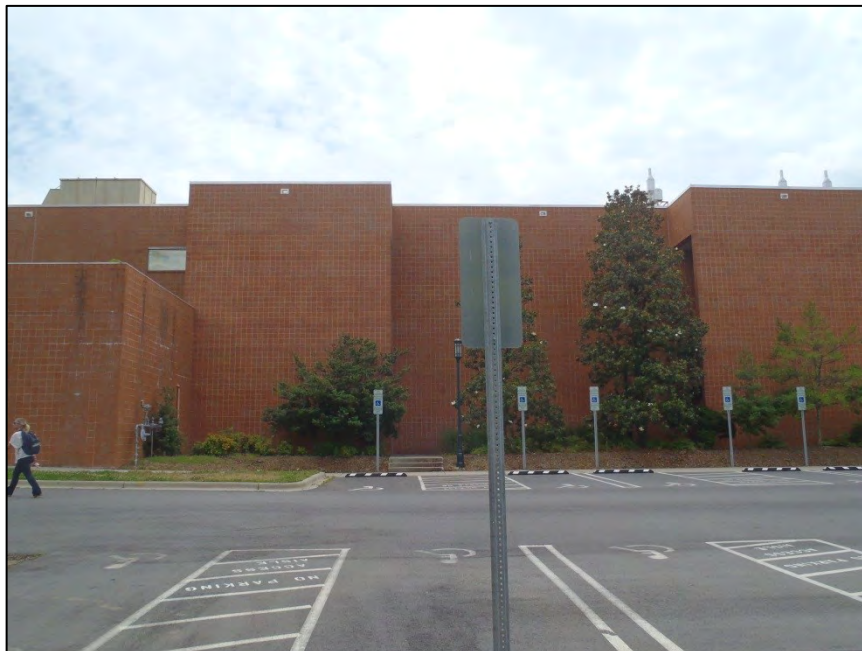
NO. 16 – PARTIAL NORTH ELEVATION
