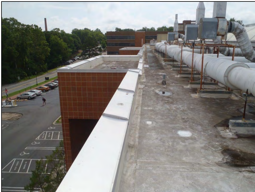
NO. 192 – ROOF VIEWS FROM THE NORTHWEST CORNER
