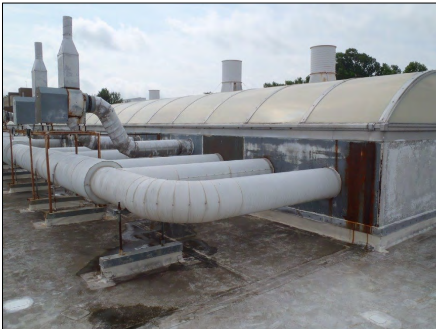
NO. 193 – ROOF VIEWS FROM THE NORTHWEST CORNER
