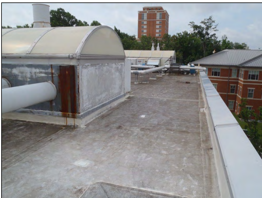
NO. 194 – ROOF VIEWS FROM THE NORTHWEST CORNER
