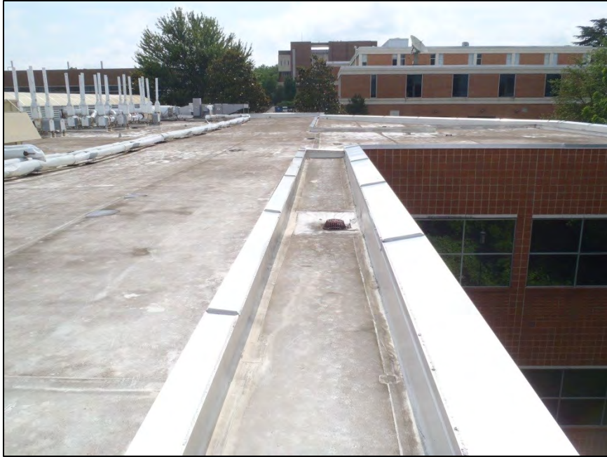
NO. 179 – ROOF VIEWS FROM THE SOUTH FACE
