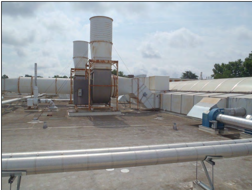
NO. 189 – ROOF VIEWS FROM THE WEST FACE
