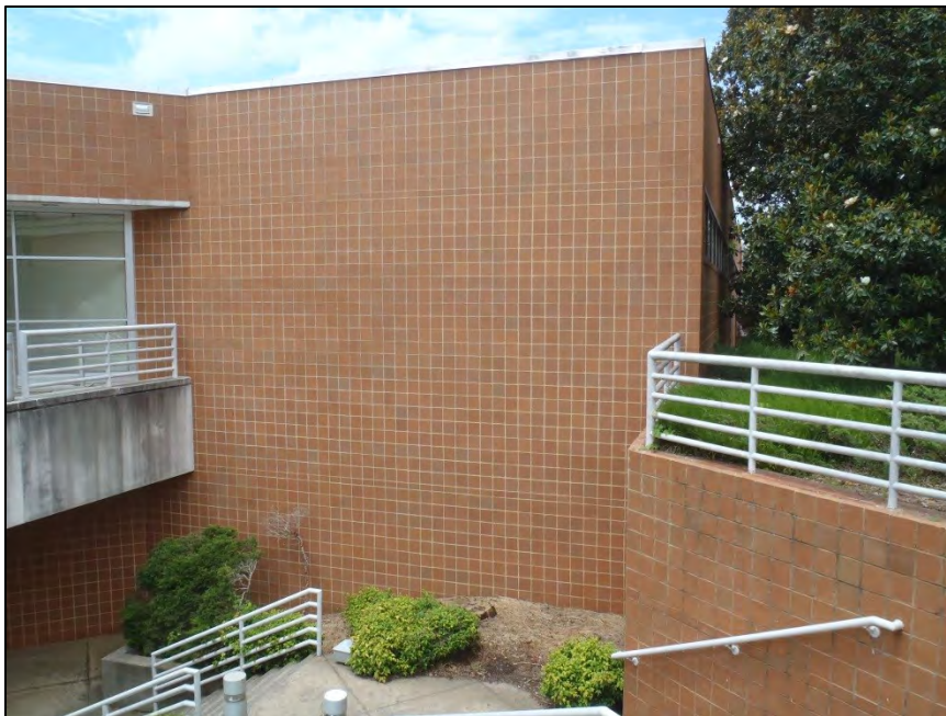
NO. 5 – PARTIAL SOUTH ELEVATION AT MAIN ENTRANCE
