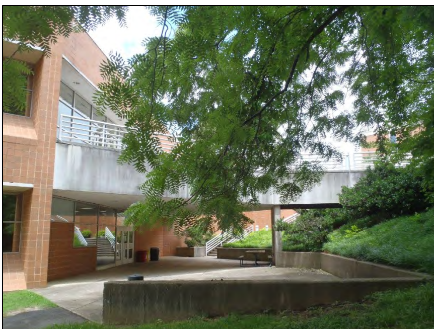
NO. 3 – PARTIAL SOUTH ELEVATION
