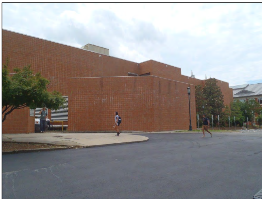
NO. 14 – PARTIAL NORTH ELEVATION
