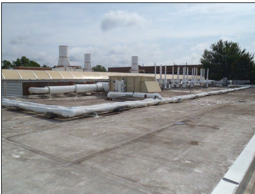
NO. 178 – ROOF VIEWS FROM THE SOUTH FACE
