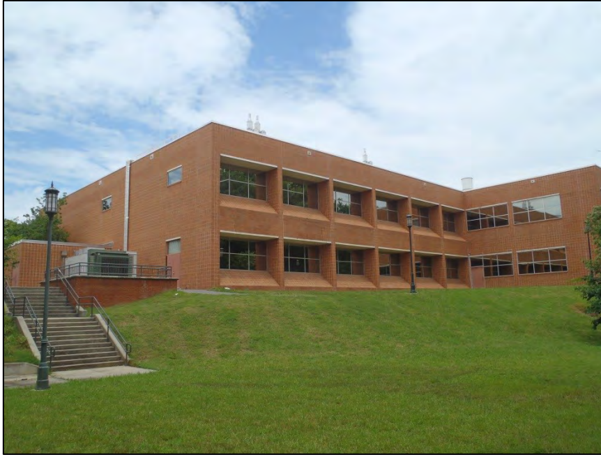
NO. 25 – PARTIAL SOUTHWEST ELEVATION
