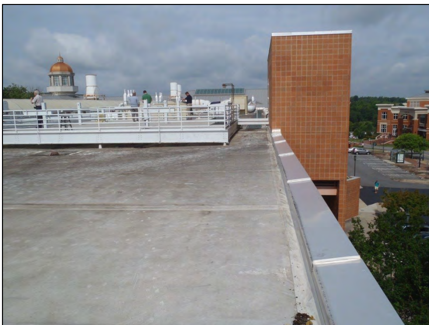
NO. 168 – ROOF VIEWS FROM THE NORTHEAST CORNER
