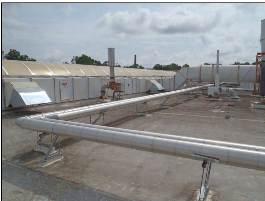
NO. 188 – ROOF VIEWS FROM THE WEST FACE
