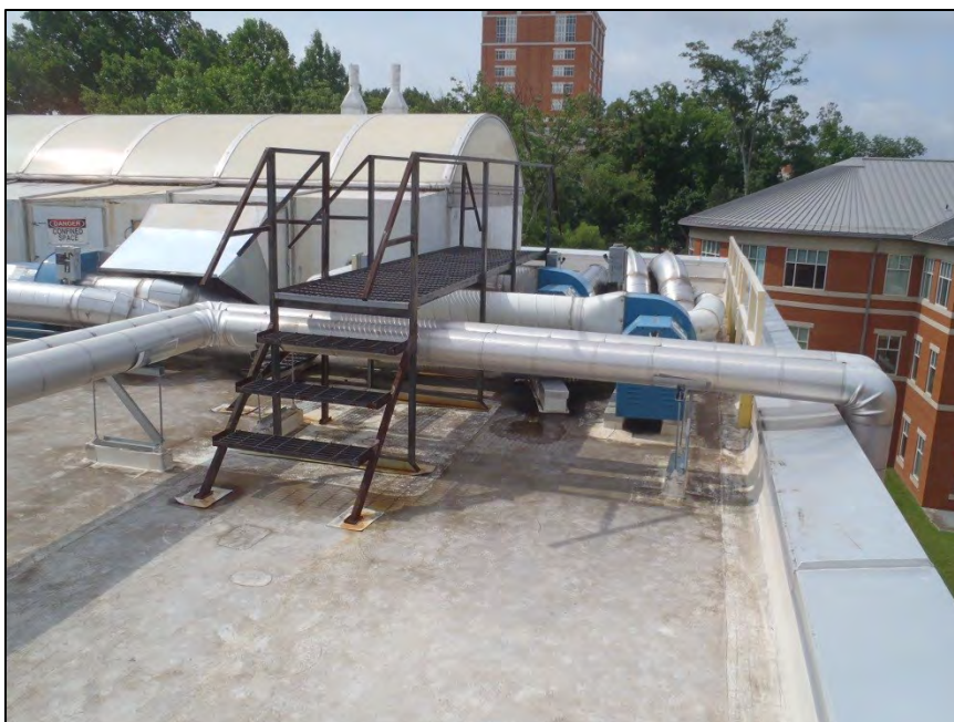
NO. 191 – ROOF VIEWS FROM THE WEST FACE
