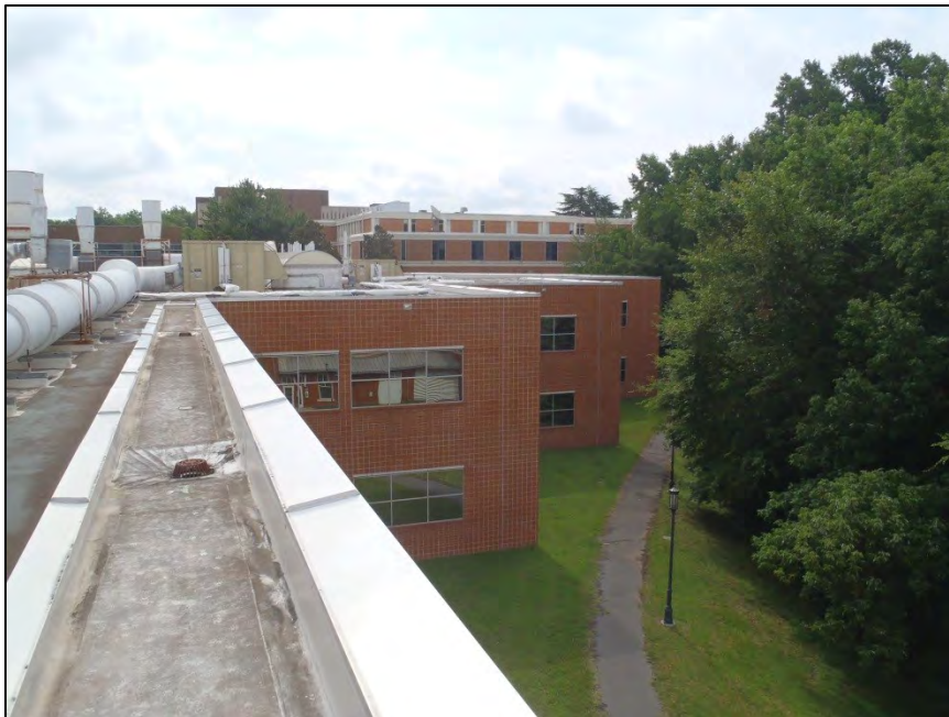
NO. 186 – ROOF VIEWS FROM THE SOUTHWEST CORNER
