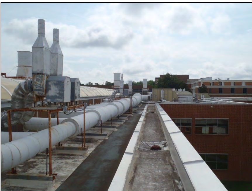
NO. 185 – ROOF VIEWS FROM THE SOUTHWEST CORNER
