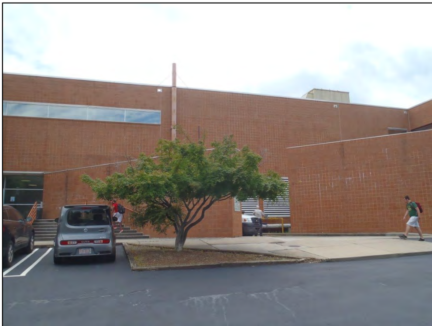
NO. 13 – PARTIAL NORTH ELEVATION
