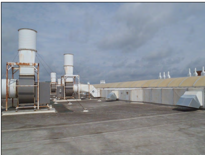
NO. 171 – ROOF VIEWS FROM THE EAST EDGE
