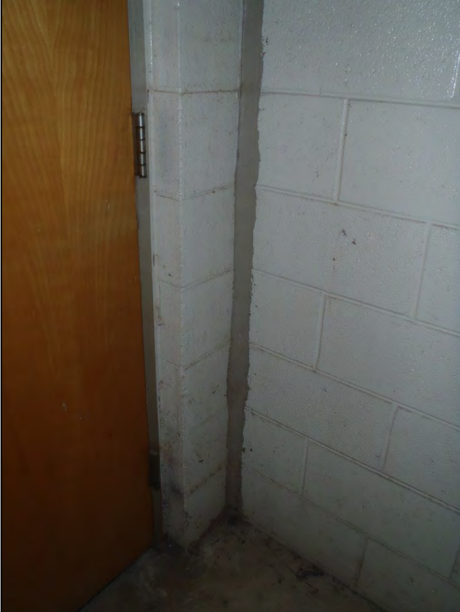
NO. 122 – FIRST FLOOR BASEMENT ADDITION – INTERIOR JOINT SEALANT
