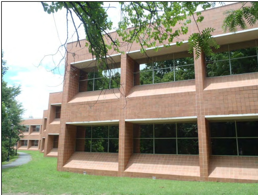
NO. 1 – PARTIAL SOUTH ELEVATION
