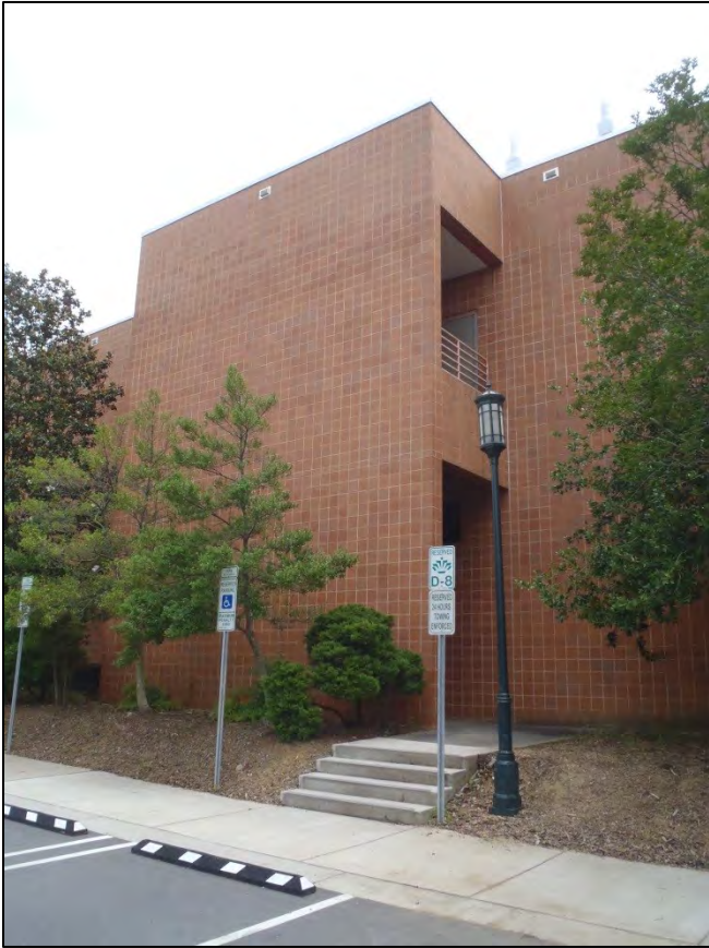
NO. 69 – NORTH ELEVATION – WEST EXTERIOR STAIRWELL
