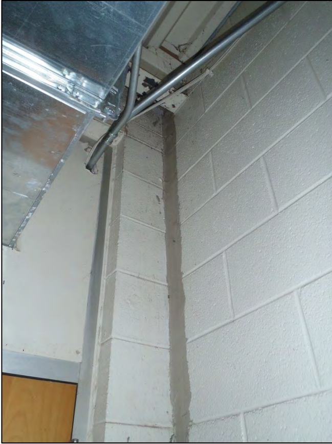
NO. 121 – FIRST FLOOR BASEMENT ADDITION – INTERIOR JOINT SEALANT
