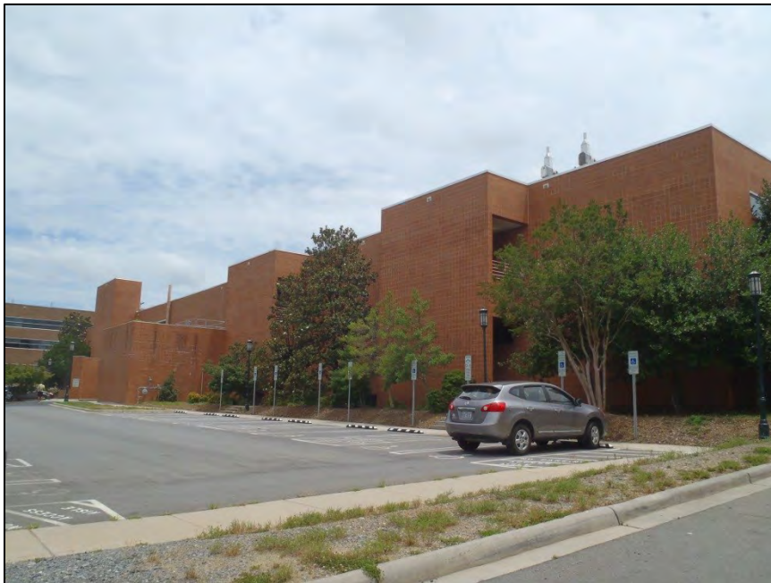
NO. 20 – PARTIAL NORTH ELEVATION
