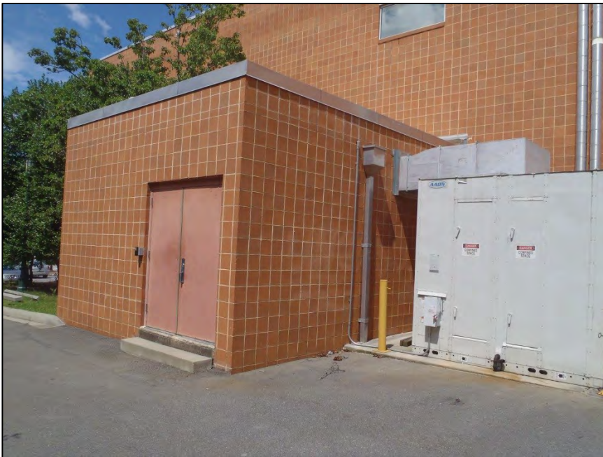
NO. 81 – WEST ELEVATION – BASEMENT ADDITION
