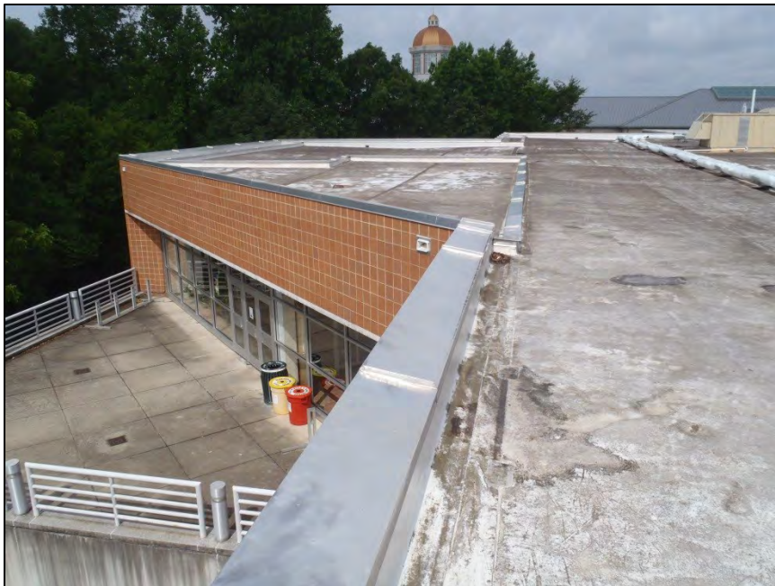
NO. 173 – ROOF VIEWS FROM THE SOUTHEAST CORNER
