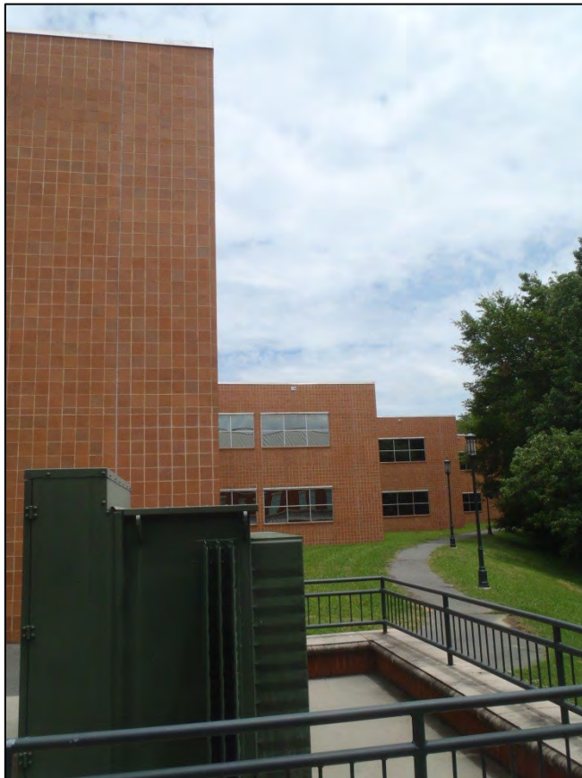
NO. 24 – PARTIAL WEST ELEVATION
