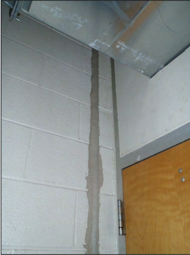
NO. 119 – FIRST FLOOR BASEMENT ADDITION – INTERIOR JOINT SEALANT
