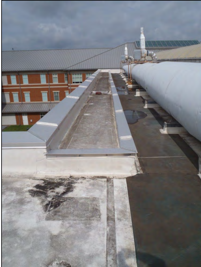
NO. 182 – ROOF VIEWS OF A SOUTH PARAPET
