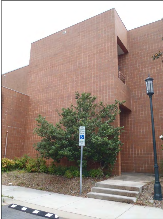
NO. 57 – NORTH ELEVATION – CENTER EXTERIOR STAIRWELL
