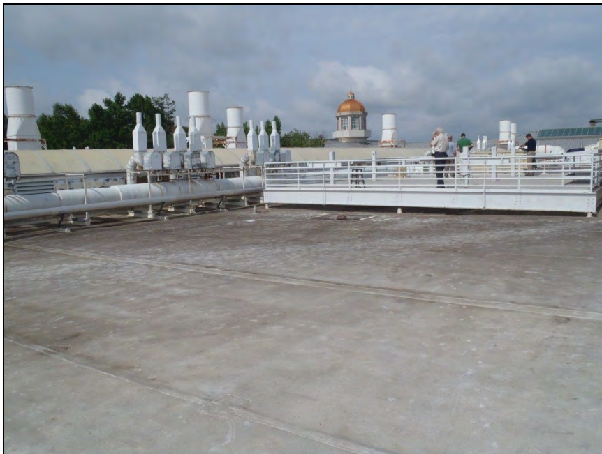
NO. 167 – ROOF VIEWS FROM THE NORTHEAST CORNER
