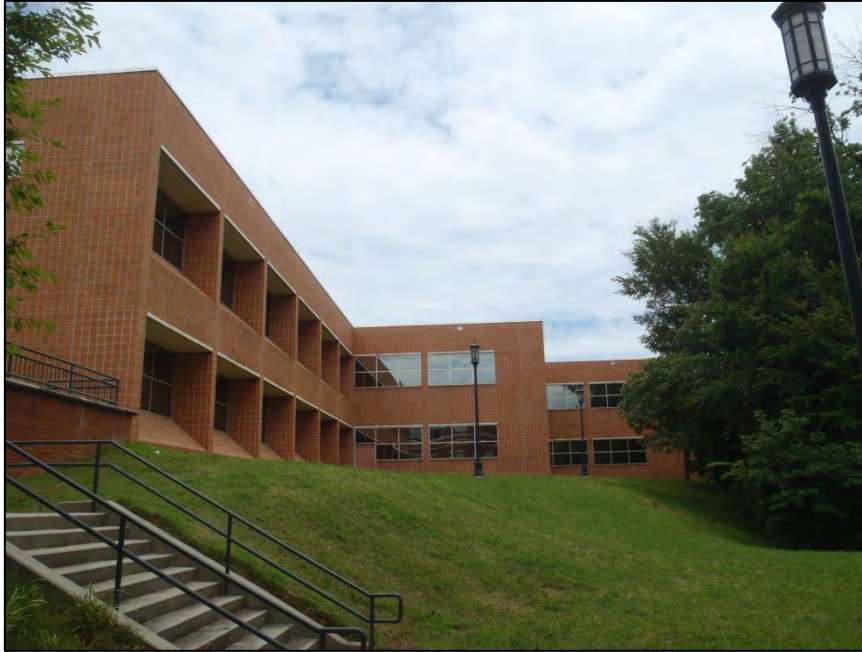
NO. 27 – PARTIAL WEST ELEVATION
