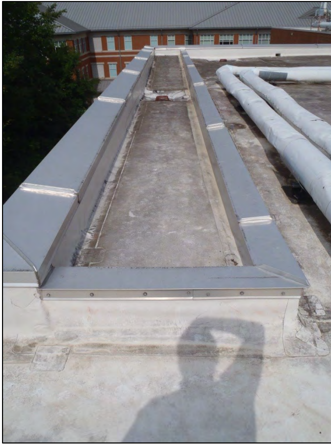
NO. 181 – ROOF VIEWS OF A SOUTH PARAPET
