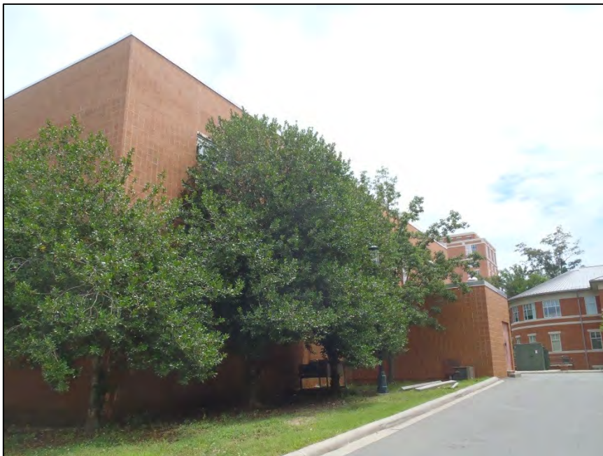
NO. 21 – PARTIAL WEST ELEVATION
