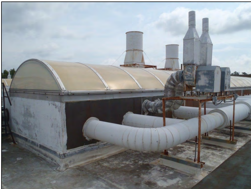
NO. 184 – ROOF VIEWS FROM THE SOUTHWEST CORNER
