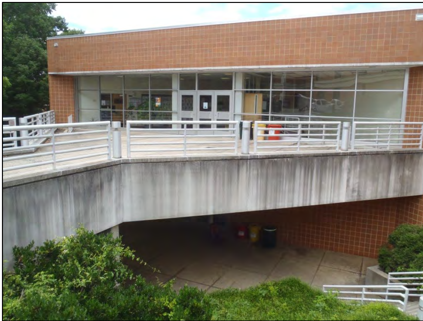
NO. 4 – PARTIAL SOUTHEAST ELEVATION AT MAIN ENTRANCE
