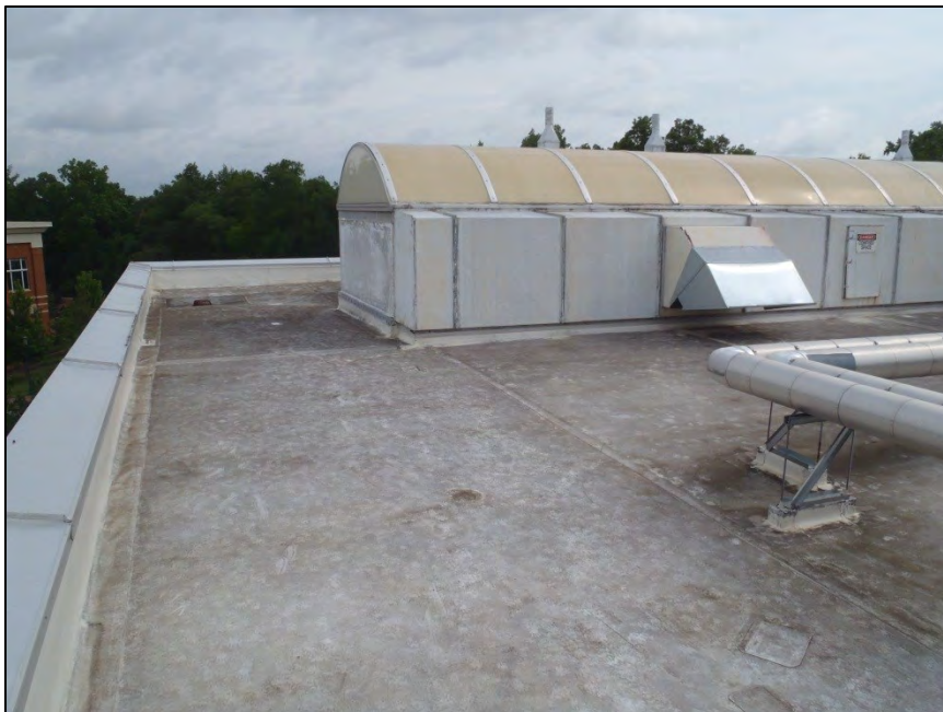
NO. 187 – ROOF VIEWS FROM THE WEST FACE
