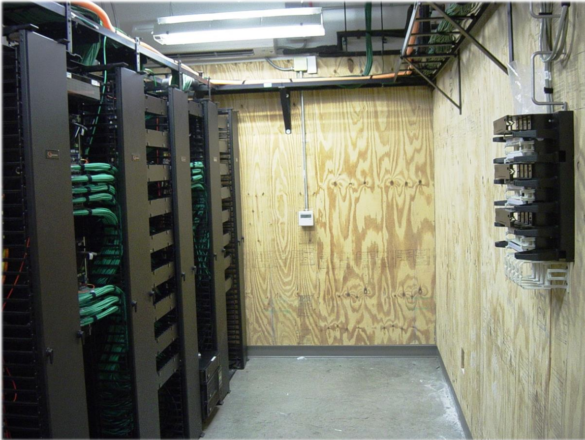
Figure 1: MDF and IDF rooms will typically be installed with a minimum of four racks with a standard equipment and patch panel configuration to be adhered to when installing network switches and patch cables. Rooms will have HVAC stand-alone units installed whenever possible and most be cooled 24X7, 365 days a year.
