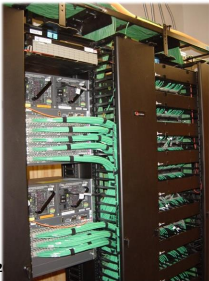
Figure 1: MDF and IDF rooms will typically be installed with a minimum of four racks with a standard equipment and patch panel configuration to be adhered to when installing network switches and patch cables. Rooms will have HVAC stand-alone units installed whenever possible and most be cooled 24X7, 365 days a year.
