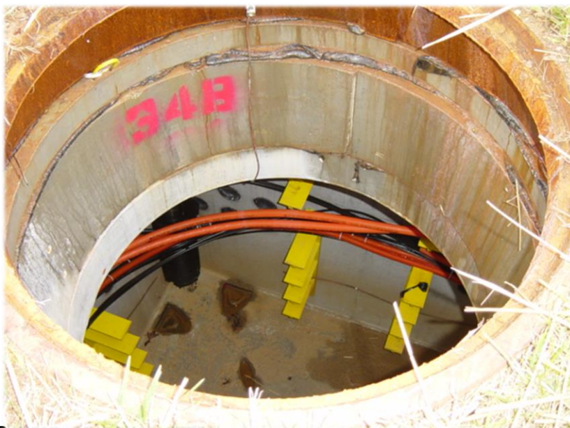
Figure 10: Telecommunications manhole and ductbanks are typically added during construction projects and when university growth requires additional conduit systems to allow for diverse fiber routes and network expansions. Extension rings are added as needed when terrain or other installation conflicts occur. Cable racking systems in manholes allow for an orderly transition of outside plant cables through the entry system.
