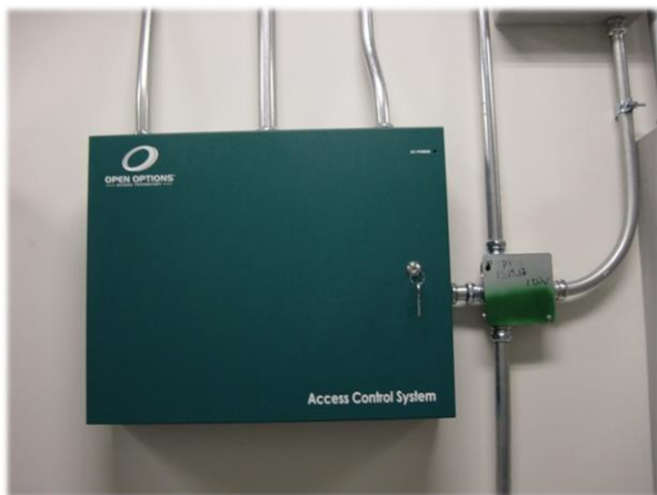
Figure 7: Access Control, Building Automation Systems, and "Pay on Foot" stations are some examples of auxiliary systems supported by the campus network. The university network also supports video surveillance, vending, and point of sales devices through hard wire and wireless access systems.
