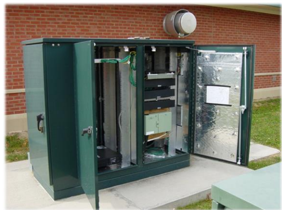
Figure 5: Wall mounted and outdoor cabinet systems will be used when dedicated data rooms are not available or when space constraints exist. These installation exceptions are coordinated during project design.
