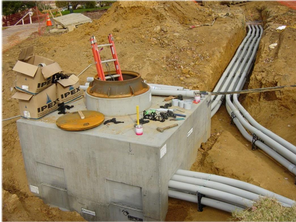
Figure 10: Telecommunications manhole and ductbanks are typically added during construction projects and when university growth requires additional conduit systems to allow for diverse fiber routes and network expansions. Extension rings are added as needed when terrain or other installation conflicts occur. Cable racking systems in manholes allow for an orderly transition of outside plant cables through the entry system.
