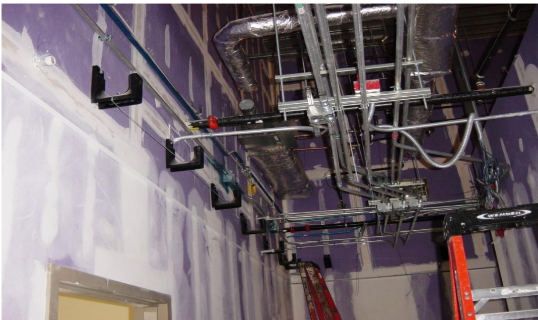
Figure 1: J-Hook cable support systems can be installed to utilize all thread or wall mounted configurations. UNCC ITS will work with the design team during advanced planning to determine the best system to be used for the new construction.
