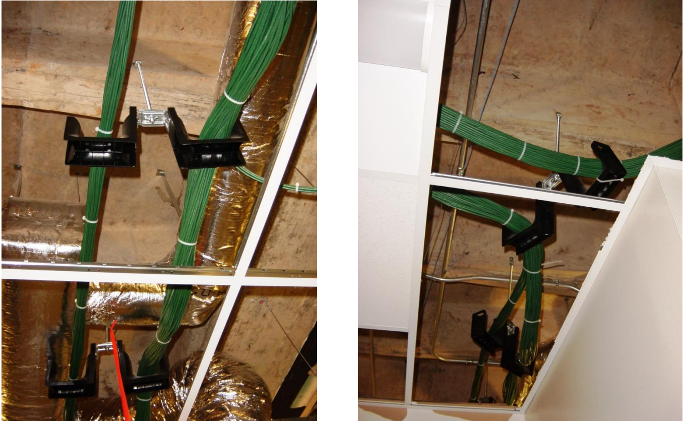
Figure 1: J-Hook cable support systems can be installed to utilize all thread or wall mounted configurations. UNCC ITS will work with the design team during advanced planning to determine the best system to be used for the new construction.
