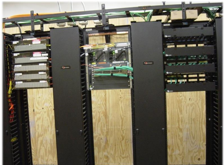
Figure 1: MDF and IDF rooms will typically be installed with a minimum of four racks with a standard equipment and patch panel configuration to be adhered to when installing network switches and patch cables. Rooms will have HVAC stand-alone units installed whenever possible and most be cooled 24X7, 365 days a year.
