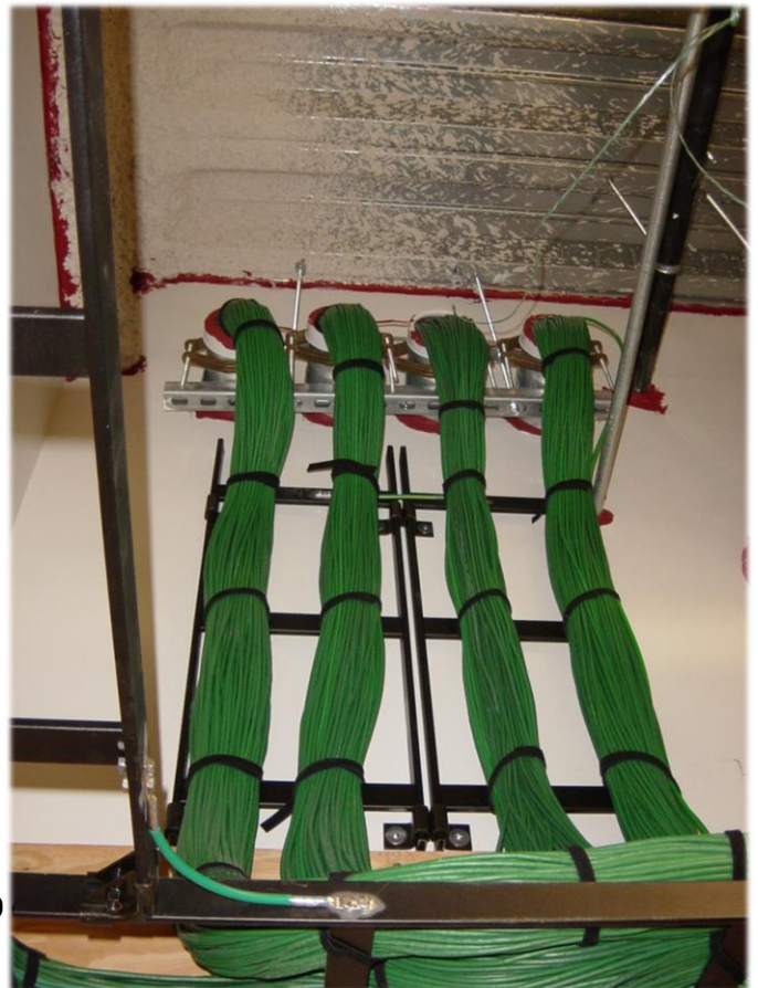
Figure 2: Fiber and copper cabling rack and wall field support systems compliment all cabling infrastructure systems used throughout campus. J-Hook and cable tray systems can be found in various building. Conveyance and pathway systems will be determined during project design.
