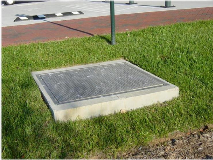
Figure 9: Telecommunications boxes (Handholes) are utilized throughout the campus and tie back to other handhole or manhole systems as necessary to facilitate cable transitions, splices and interconnects between equipment and buildings. Local carriers such as AT&T, Time Warner, and Windstream enter our campus through a joint ductbank and handhole system that connect through conduits back to the university manhole as seen below.
