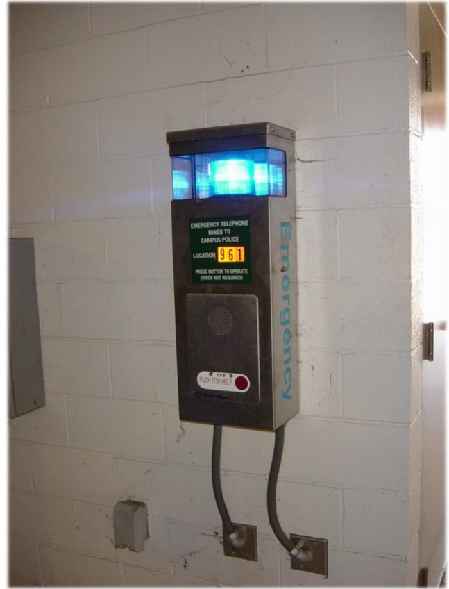
Figure 6: Emergency Phones are installed throughout the campus. Code Blue Pole phones (standard) replace older Yellow Box phones. Wall mounted blue phones can be found in most parking decks.
