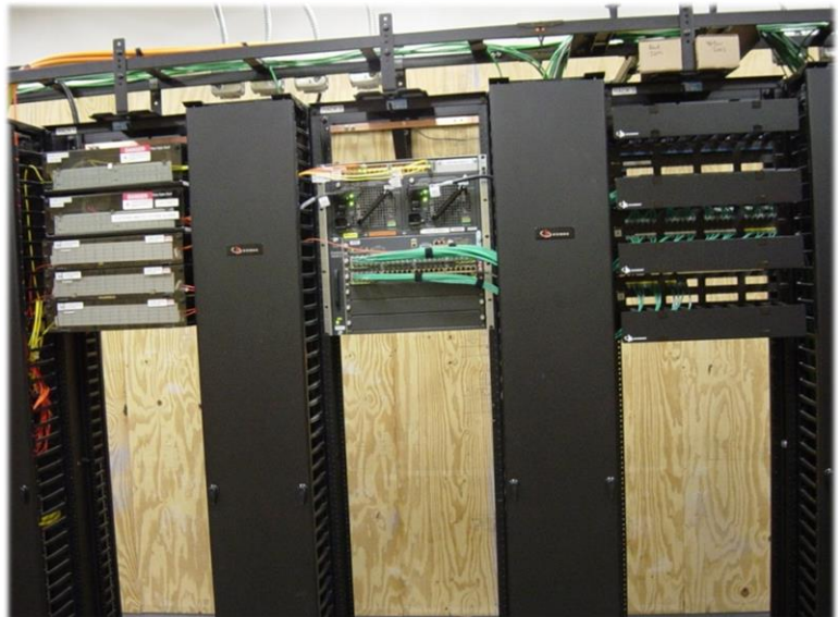
Figure 1: MDF and IDF rooms will typically be installed with a minimum of four racks with a standard equipment and patch panel configuration to be adhered to when installing network switches and patch cables. Rooms will have HVAC stand-alone units installed whenever possible and must be cooled 24X7, 365 days a year.
