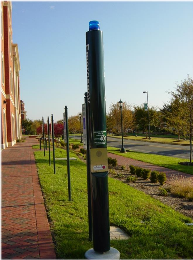
Figure 6: Emergency Phones are installed throughout the campus. Code Blue Pole phones (standard) replace older Yellow Box phones. Wall mounted blue phones can be found in most parking decks.
