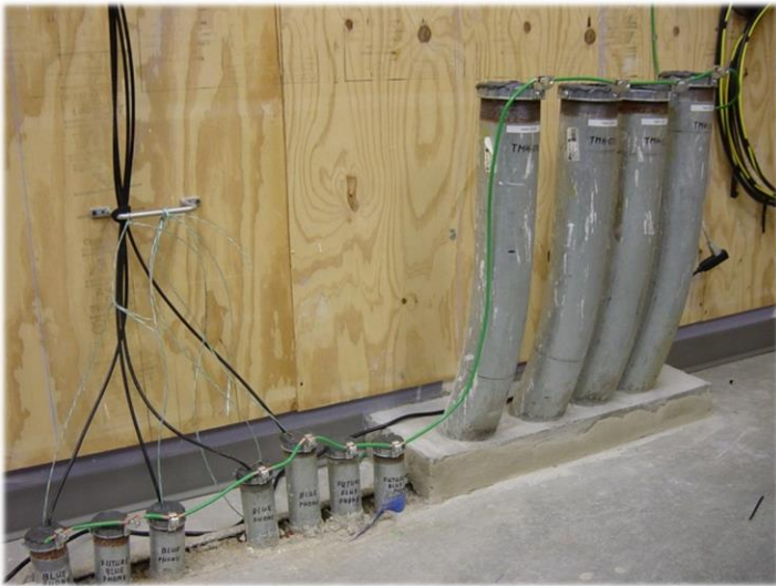
Figure 4: Conduits entering from below slab should be labeled and bonded. Main Ground Bar systems will be installed in each MDF and IDF room.
