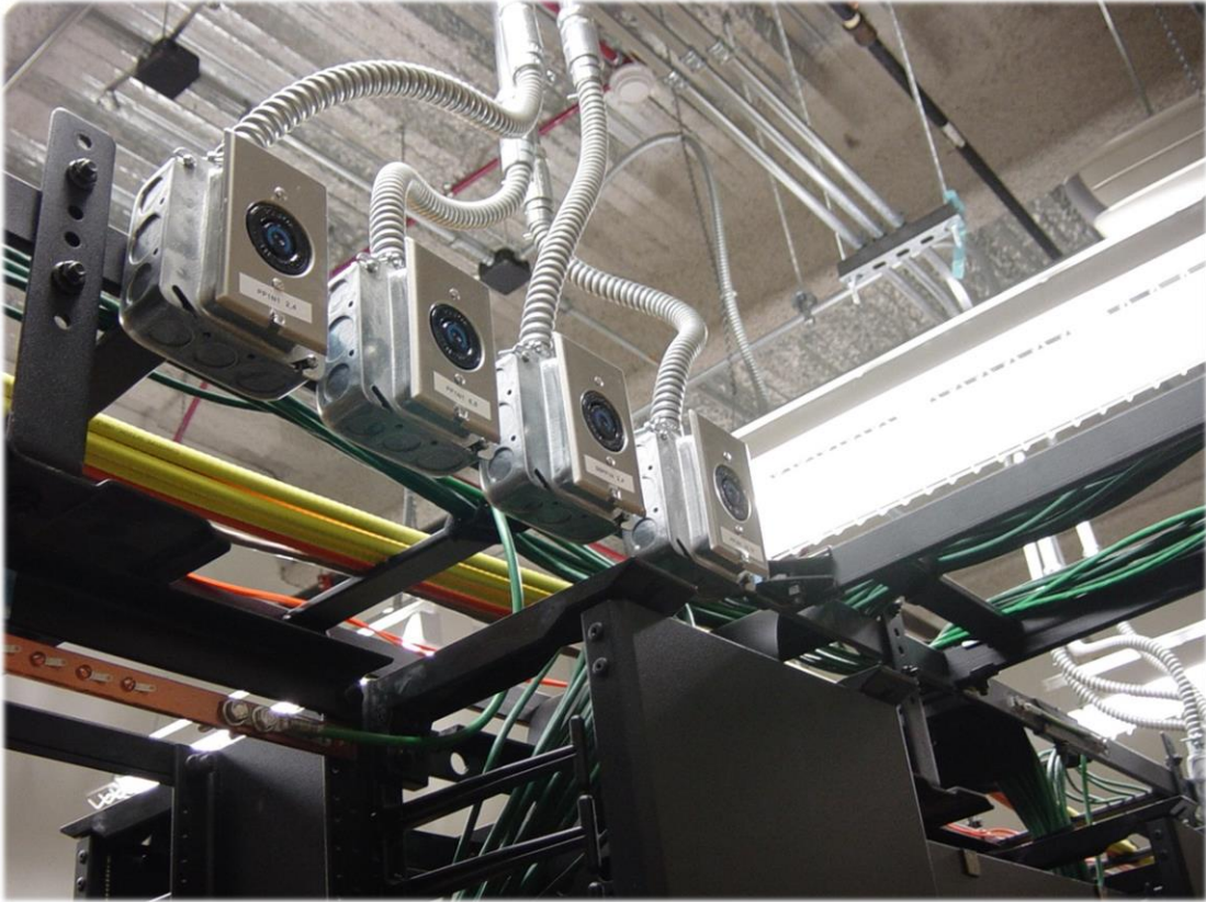
Figure 3: Outlet types vary in the MDF and IDF telecommunications rooms. Locations for these outlets will be determined at the beginning of the project during the construction design meetings. Typically, all outlets required will be installed above the equipment racks and in the rear of the rack system.
