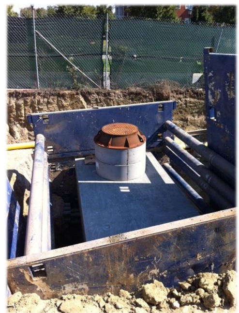
Figure 10: Telecommunications manhole and ductbanks are typically added during construction projects and when university growth requires additional conduit systems to allow for diverse fiber routes and network expansions. Extension rings are added as needed when terrain or other installation conflicts occur. Cable racking systems in manholes allow for an orderly transition of outside plant cables through the entry system.
