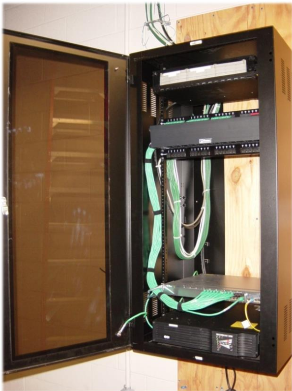
Figure 5: Wall mounted and outdoor cabinet systems will be used when dedicated data rooms are not available or when space constraints exist. These installation exceptions are coordinated during project design.
