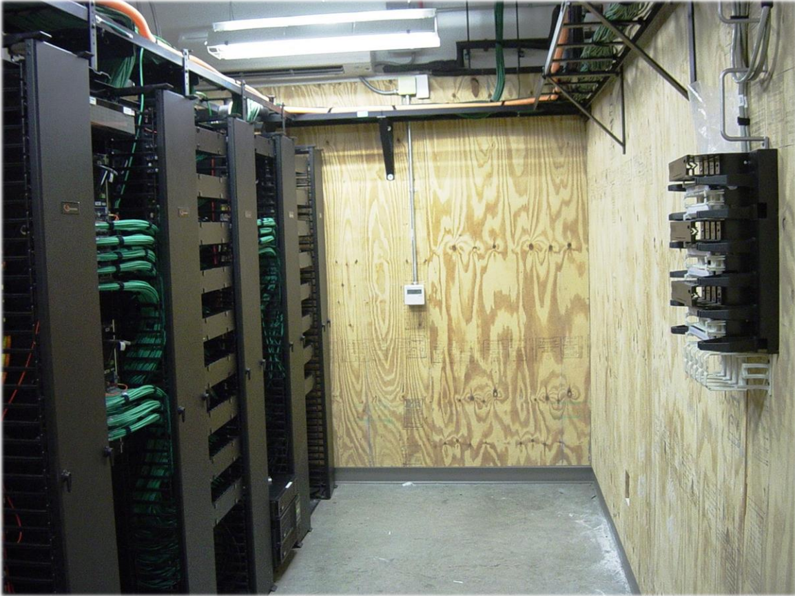
Figure 1: MDF and IDF rooms will typically be installed with a minimum of four racks with a standard equipment and patch panel configuration to be adhered to when installing network switches and patch cables. Rooms will have HVAC stand-alone units installed whenever possible and must be cooled 24X7, 365 days a year.
