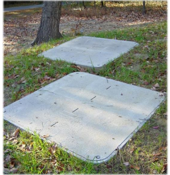
Figure 9: Telecommunications boxes (Handholes) are utilized throughout the campus and tie back to other handhole or manhole systems as necessary to facilitate cable transitions, splices and interconnects between equipment and buildings. Local carriers such as AT&T, Time Warner, and Windstream enter our campus through a joint ductbank and handhole system that connect through conduits back to the university manhole as seen below.
