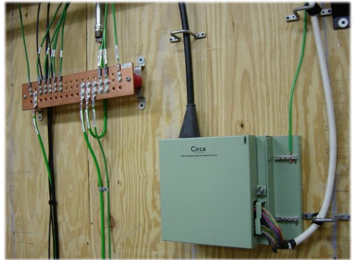
Figure 4: Conduits entering from below slab should be labeled and bonded. Main Ground Bar systems will be installed in each MDF and IDF room.
