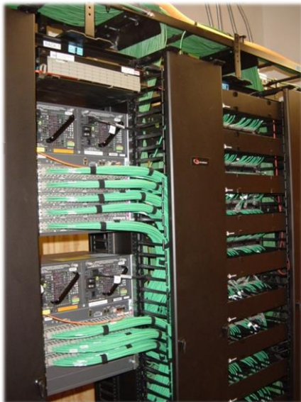
Figure 1: MDF and IDF rooms will typically be installed with a minimum of four racks with a standard equipment and patch panel configuration to be adhered to when installing network switches and patch cables. Rooms will have HVAC stand-alone units installed whenever possible and must be cooled 24X7, 365 days a year.
